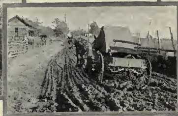
Typical Spring condition of soft-surfaced roads
